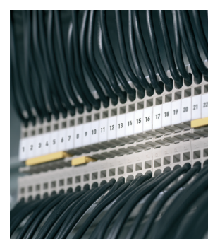
Assembled and wired terminal rails ready to be installed
