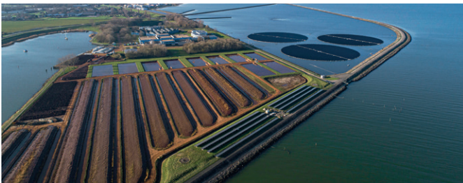
Floating dynamic solar park Dynamic solar islands
